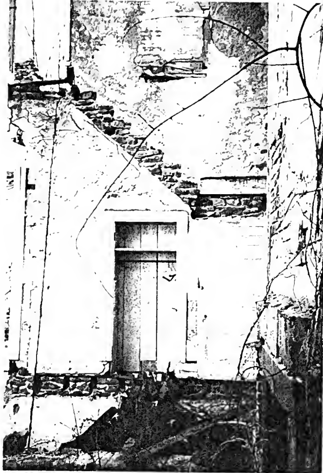
Figure 21: Interior wall of Wetherill addition showing imprint of second story stair over previous central hall.
